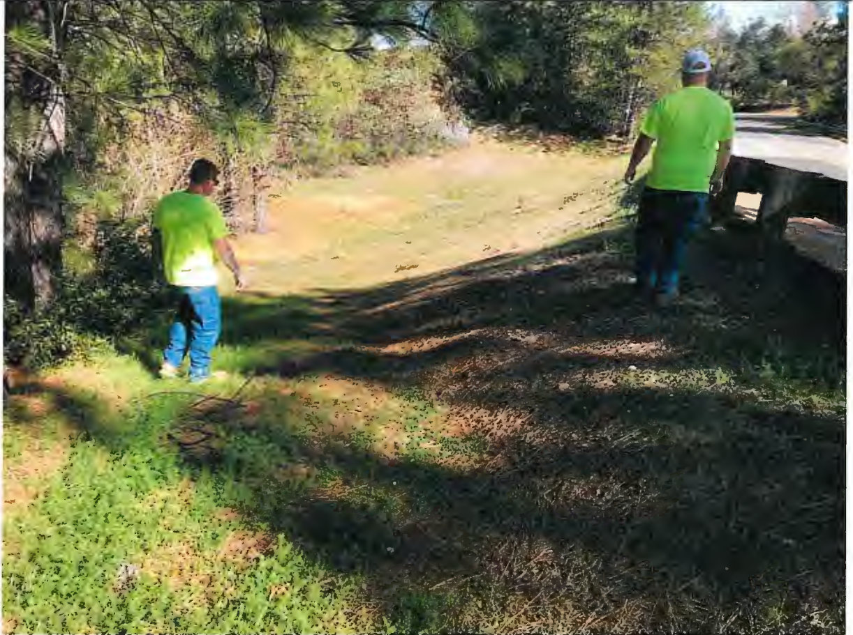
5. Main Dam downstream face observed from left side. Good vegetation control.
