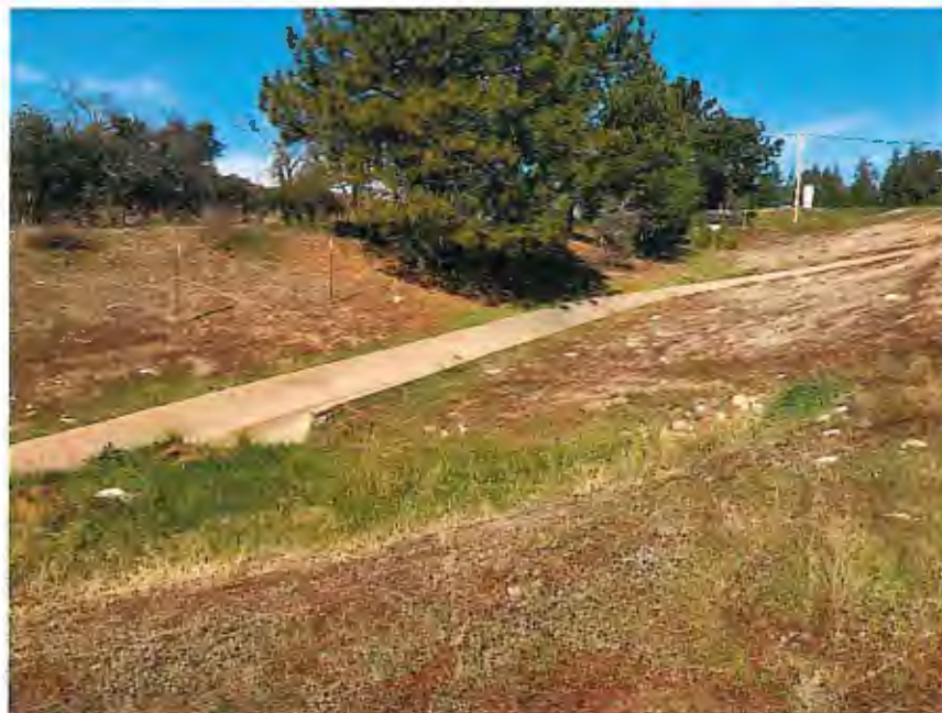
4. Concrete lined spillway channel.
