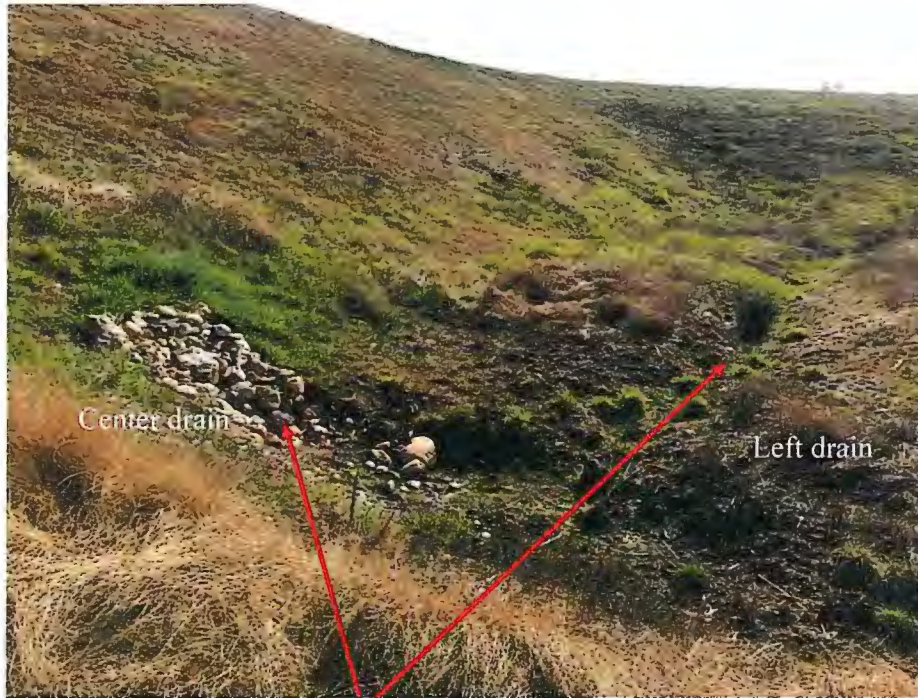
3. View of two drains at the toe of the West Dike.
