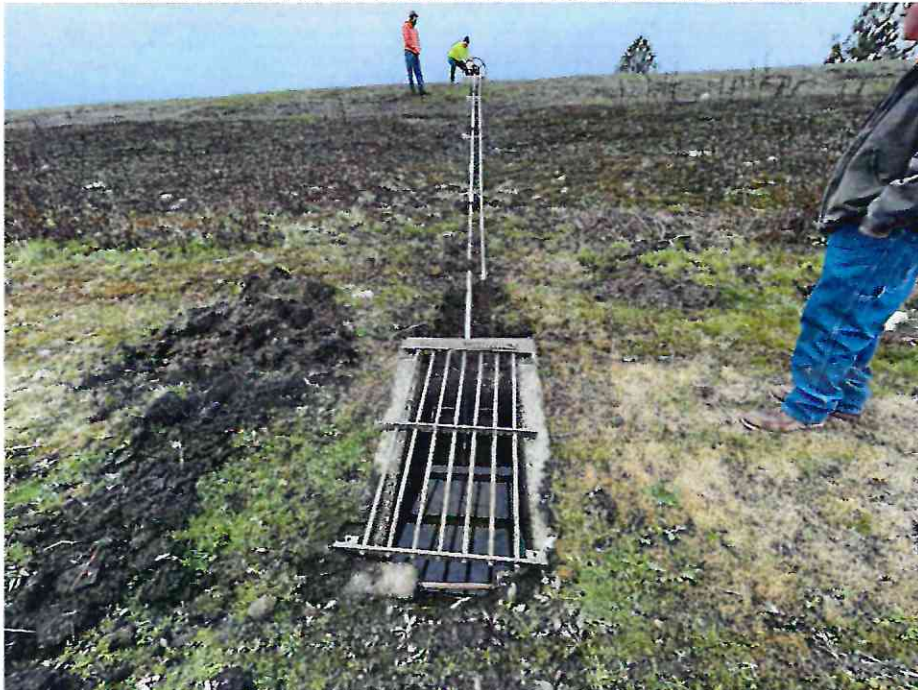
Photo 6: View of the upstream slide gate inlet looking downstream.
