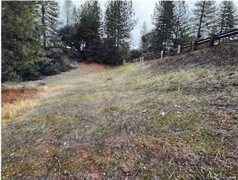
Photo 5: View of the downstream face of the Main Dam.
