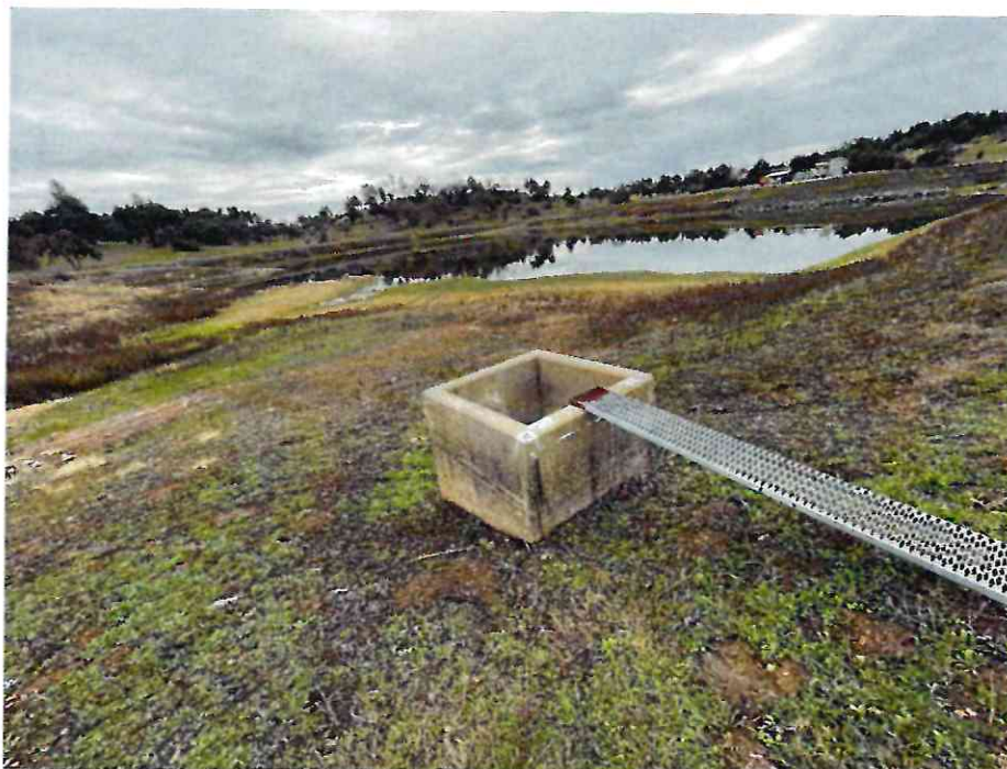
Photo 7: View of the spillway approach and drop inlet.
