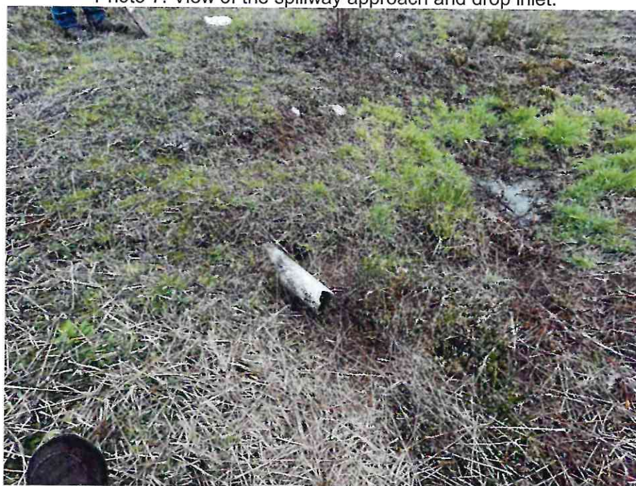
Photo 8: View of the left drain at the toe of the West Dike.
